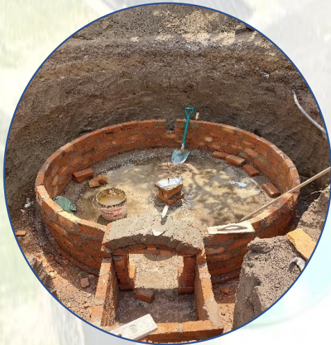
Construction of Fixed Dome Biogas at Ngarantoni
